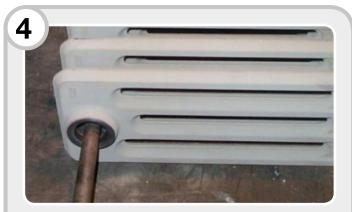
**IMPORTANT:** At this stage only rotate the nipple by one turn then repeat this operation with the other nipple. Repeat both of these operations in turn, gradually pulling the two radiator assemblies together, ensuring they are pulled up in parallel.
