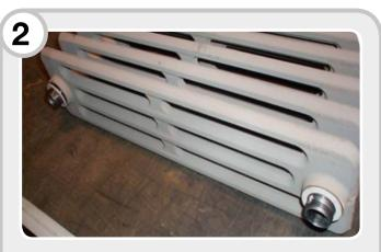
Note: **Smooth end of nipple = right hand thread**, look into the radiator header, the prior nipples edge will help you orientate your jointing nipple correctly.
