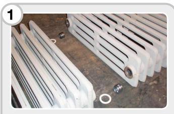
Place the radiator sections to be joined onto a clean, firm and flat surface, ensuring that the machined faces and internal threads are perfectly flat and clean.
