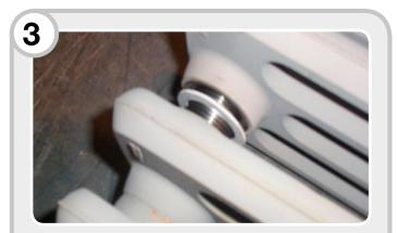
Slide the second radiator block up to the nipples, ensuring that the section/thread orientations are all correct.
